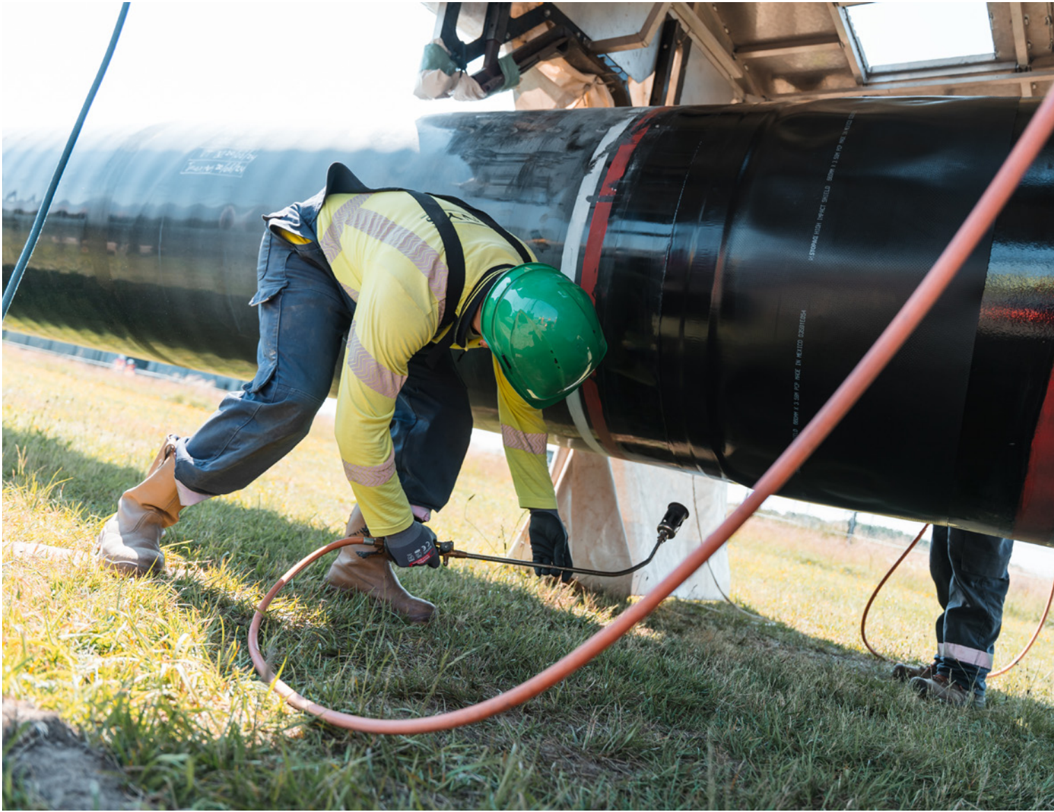
A worker putting the finishing touches on the welding process of two pieces of pipeline as part of the Porthos carbon transport and storage project, required for low-carbon hydrogen production.
