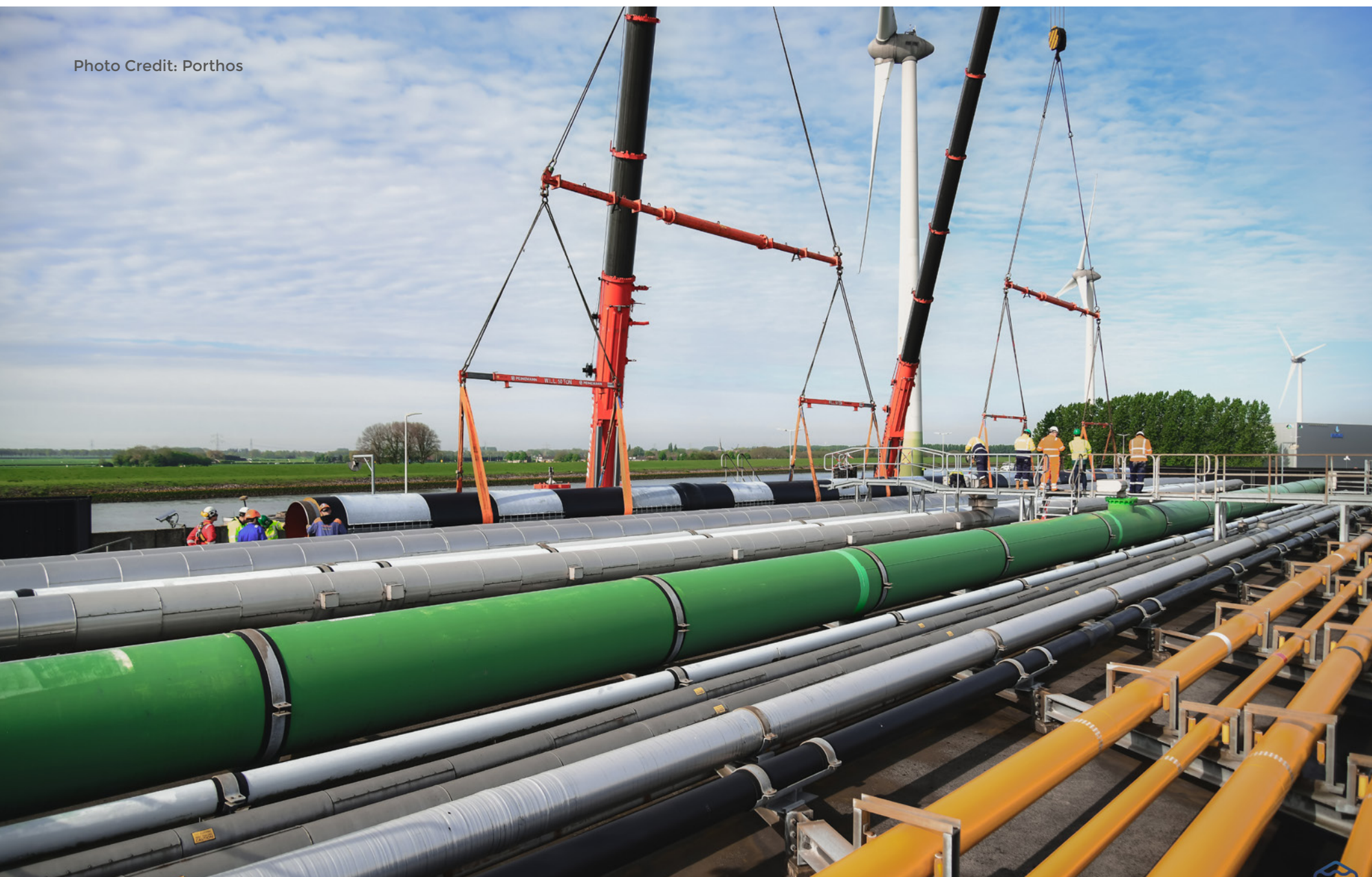
Lifting the pipe on the Welplaatviaduct.
